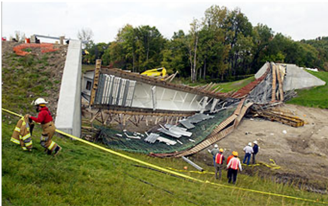
Figure 1.3 Collapse of pedestrian bridge near Marcy, New York (Utica Observer-Dispatch)
